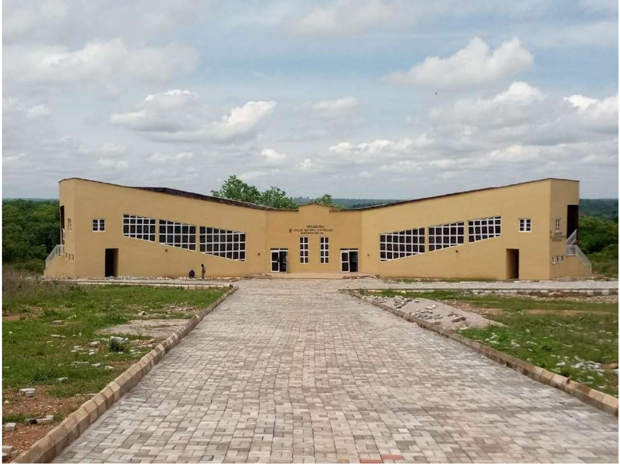
Tetfund 2018 High Impact Twin Lecture Hall
