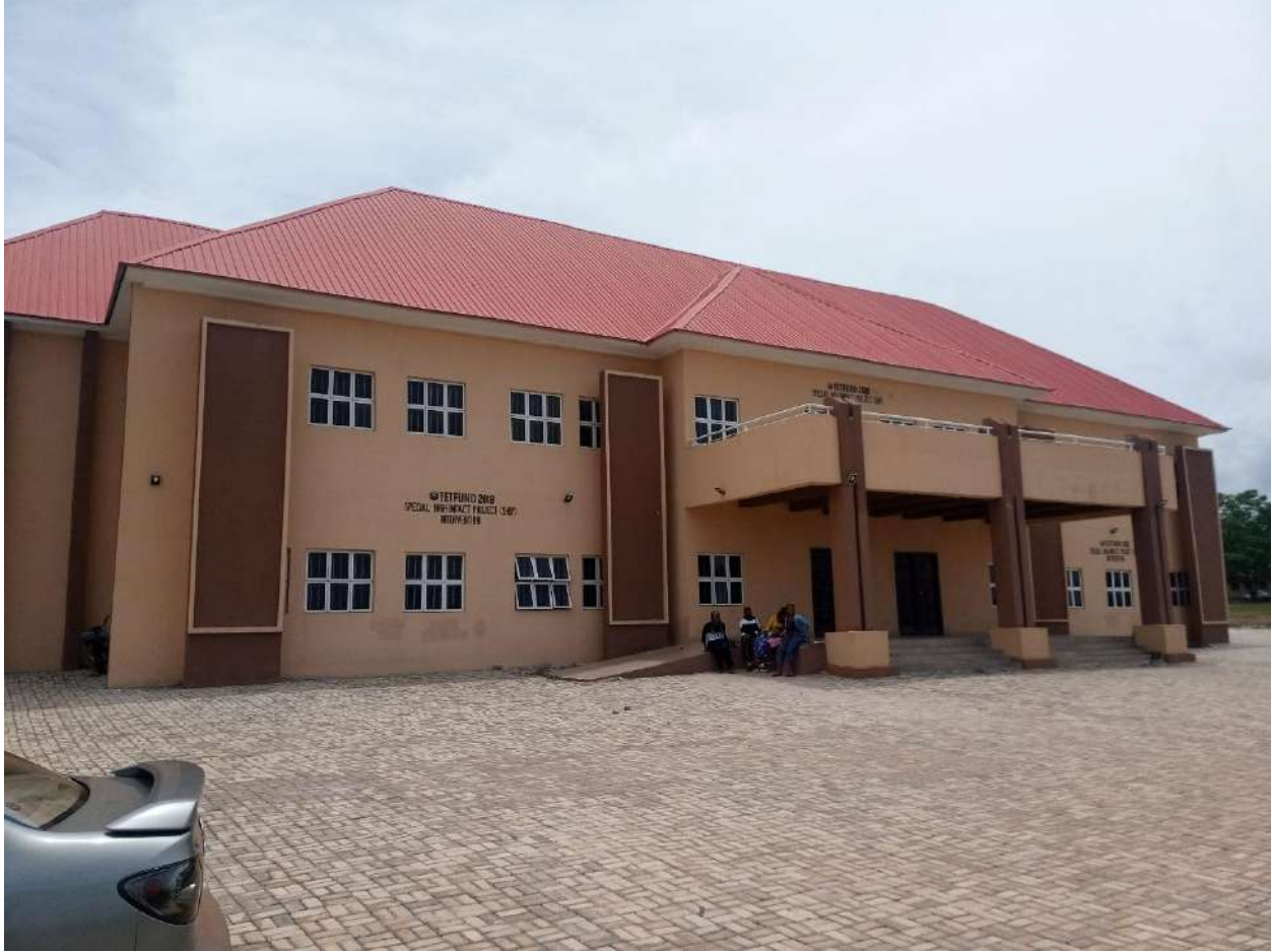
Tetfund 2018 High Impact Lecture Rooms and Offices
